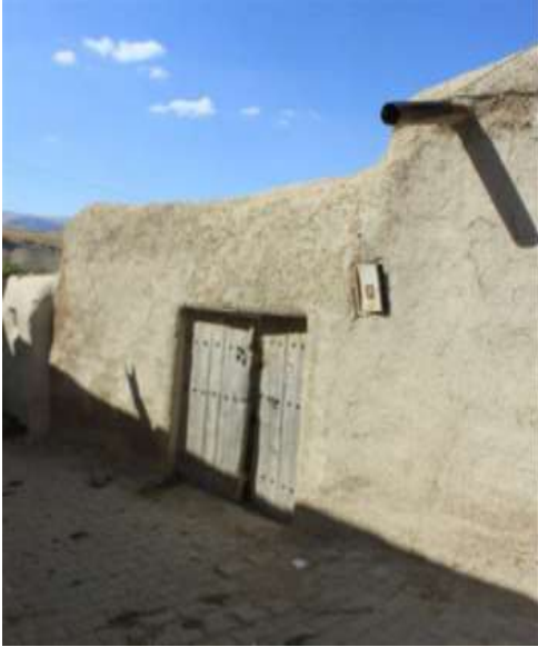
Foto 3b. Güneybatı cephe (Photo 3b. Southwest front)
