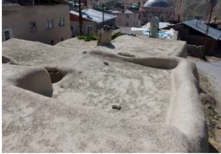
Foto 3h. Toprak dam (Photo 3h. Soil roof)
