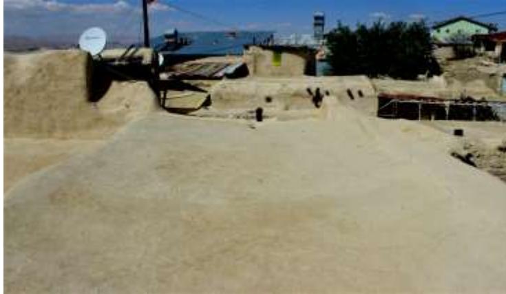
Foto 2j. Toprak dam (Photo 2j. Soil roof)
