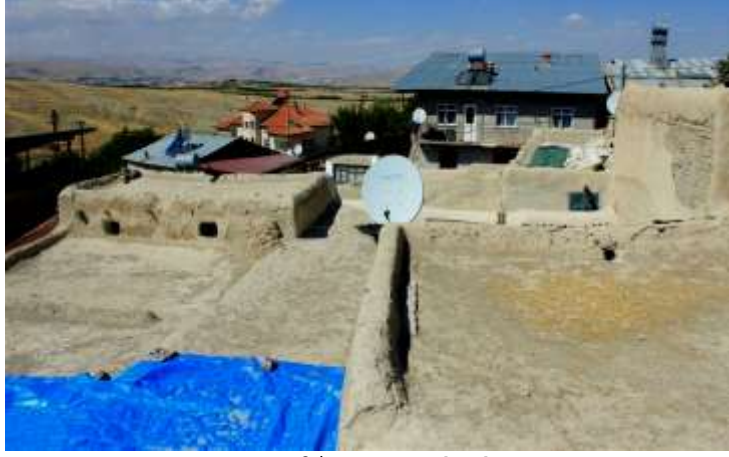
Foto 2i. Toprak dam (Photo 2i. Soil roof)
