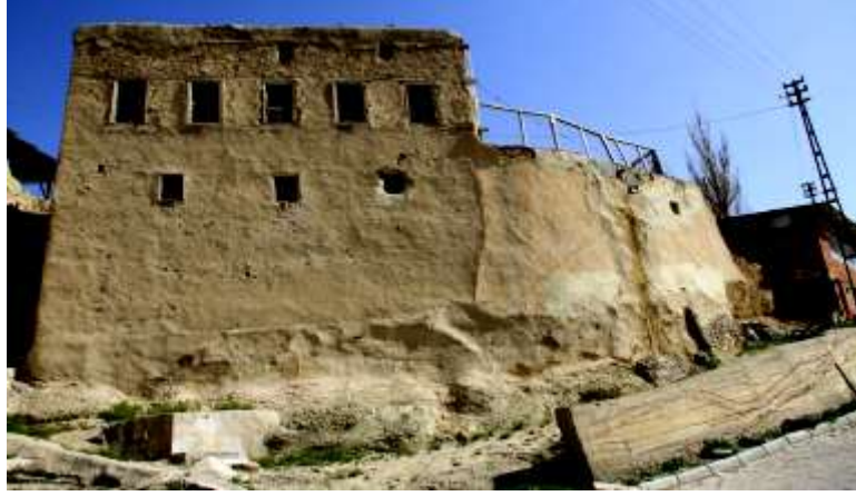
Foto 1b. Güney cephe (Photo 1b. South front)
