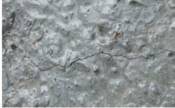
Resim 2. Bünyesel-hidratasyon-otojen (autogenous) rötire örneği [85] (Photo 2. Example of structural-hydration-autogenous shrinkage)
