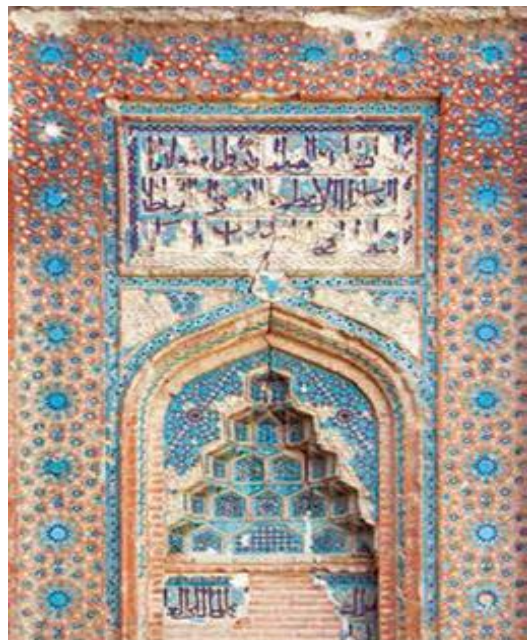
Image 11. brick working of glazed tiles in Ghafarieh dome (writers)
