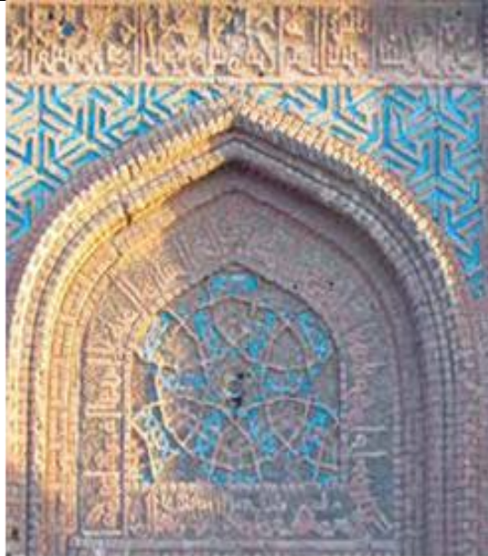
Image 10. Girih tiles with the incorporation of brick and tile in Ghafarieh dome (writers)
