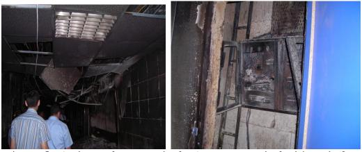
The fact that both electrical wiring and piping for vesicant gases such as oxygen, accelerating the burning process, were installed in the same ducting shaft with the dimensions of 165x65 cm is another important factor which contributed to the spread of the fire to the intensive care center which was located on the 3rd floor. Moreover the doors of fire escape stairs were locked for security purposes delaying vertical evacuation.
